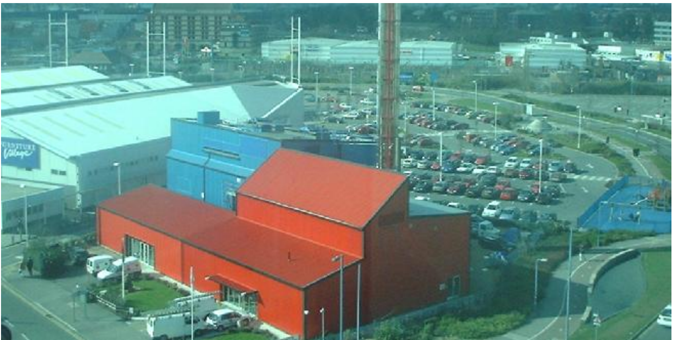
Figure 1. Utilicom's Southampton Geothermal Heating Company's facilities - West Quay, Southampton.
